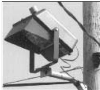
These fixtures are mounted on wooden utility poles. Many of these lights are very noticeable along major and minor roadways because they have been installed quite inappropriately. They are a source of considerable glare and unnecessary light spilling into adjacent property. The photo at far left shows such a fixture. The next photo shows a properly installed fixture. Note how it is aimed more downward and has a shield to prevent light-spillage.
